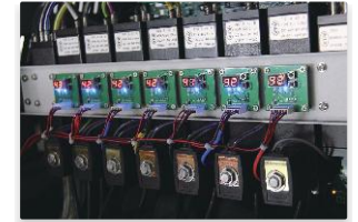
Negative Pressure System
