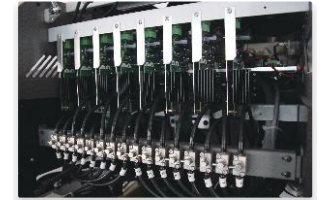
Negative Pressure System
